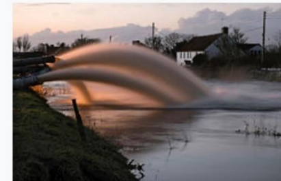
Emergency pumps were brought in to drain the Somerset levels.
